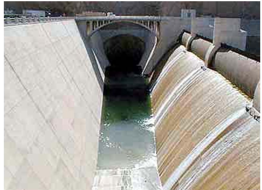
Hoover Dam side channel spillway
