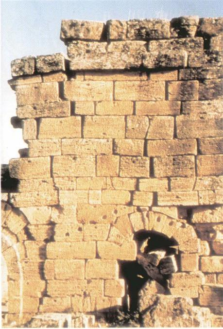
**Fig. 12.** Fissures cutting the walls of part of the Northern Baths, a monument built of bedded travertine blocks. Fissuring is a characteristic form of damage in dry masonry walls shaken during an earthquake.
