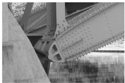
In particular, if the arch has a parabolic shape and it is subjected to a uniform horizontally distributed vertical load, then only compressive forces will be resisted by the arch. Under these conditions the arch shape is called a funicular arch because no bending or shear forces occur within the arch.
