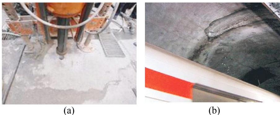
Fig. 3a, b: Pierced tube of the Taksim-Levent subway
