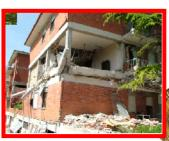
According to theoretical results and to the experiences gained from examining the performances of RC structures after seismic events it was decided to design a local FRP based strengthening intervention on partially confined beam columns joints to quickly strengthen the RC building of L'Aquila
