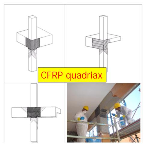
shear capacity increase of beam – column joint panel: the shear increase of beam column joint can be achieved through the application of composites with fibers placed along the principal tensile stresses (i.e. quadriaxial FRP laminates) for a corner joint and for an exterior one
