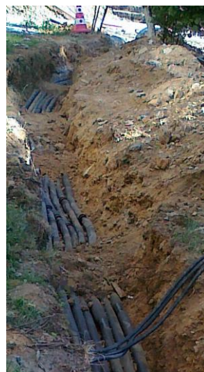
Figure 6: Connections between Borehole and laboratory before close the trench
