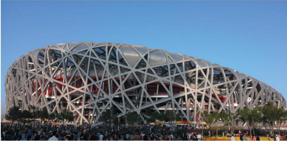
Figure 2.2 The perimeter steel structure wraps around the inner concrete bowl (Arup).
