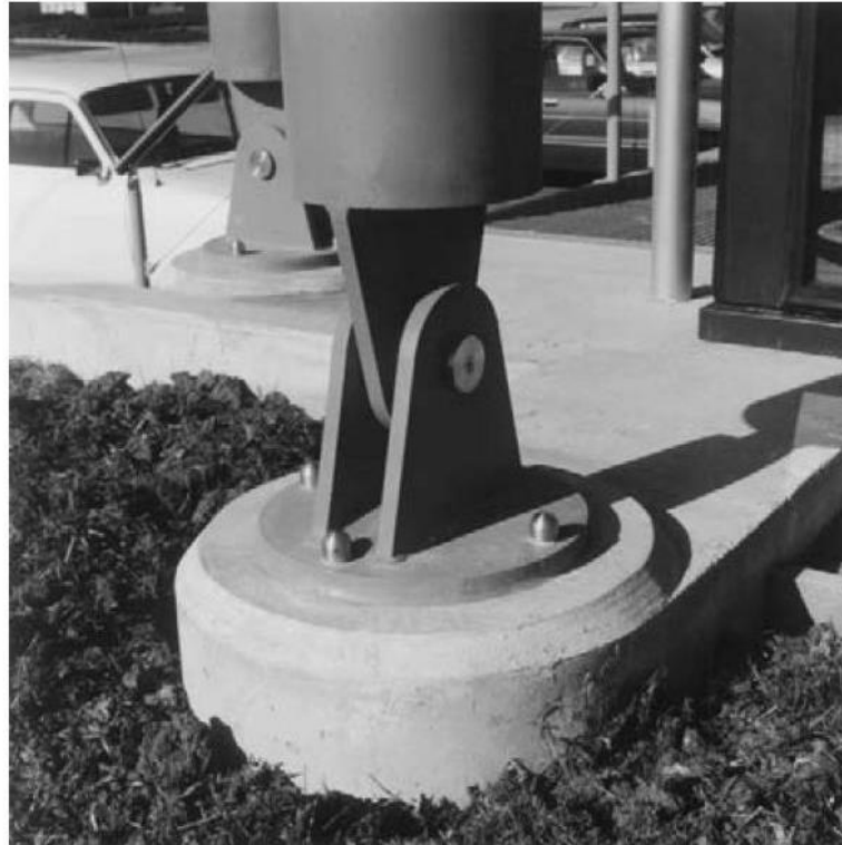
6.13 Typical pinned connection to a foundation
