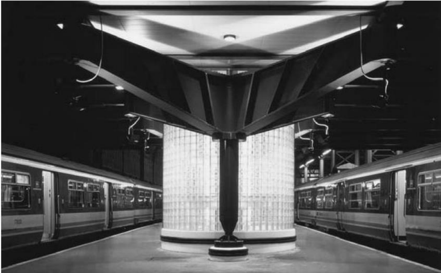
1.8 Operations Centre at Waterloo, London, showing a fabricated cantilever beam supporting a walkway (architect: Nicholas Grimshaw & Partners)
