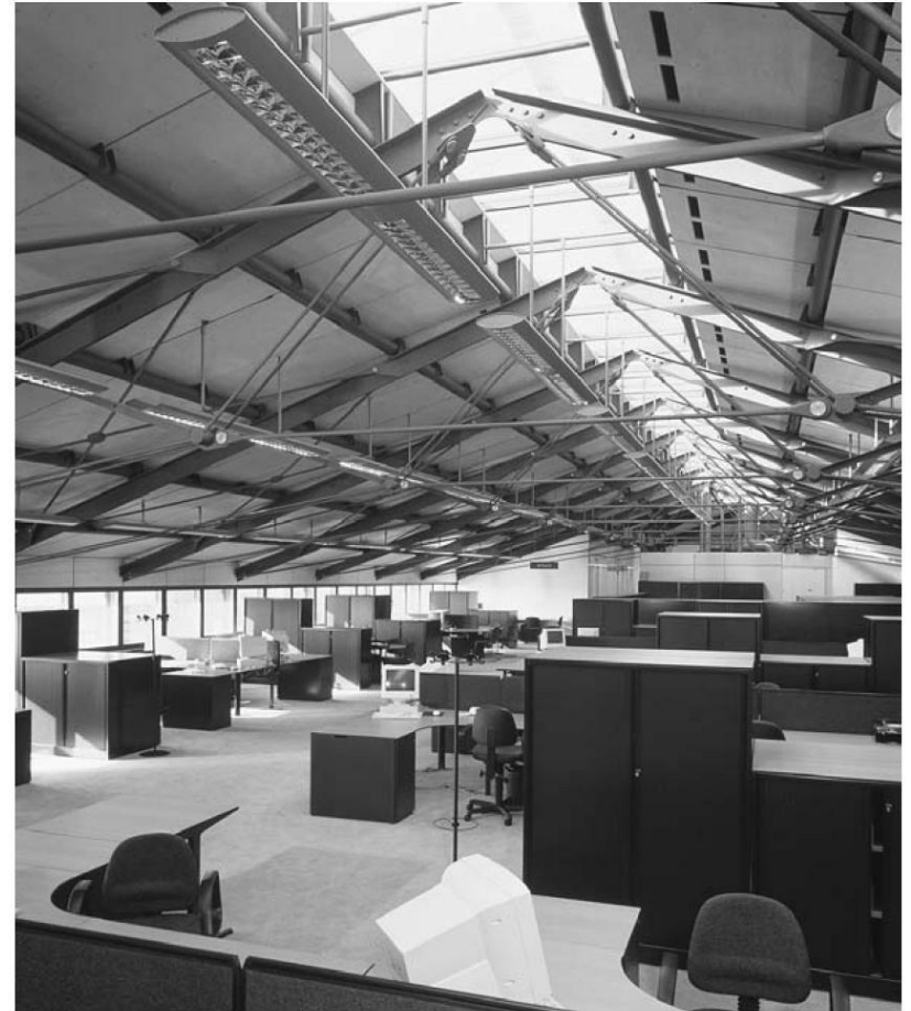
1.7 Inland Revenue Headquarters, Nottingham, showing truss details which provide interest and articulation (architect: Michael Hopkins and Partners)
