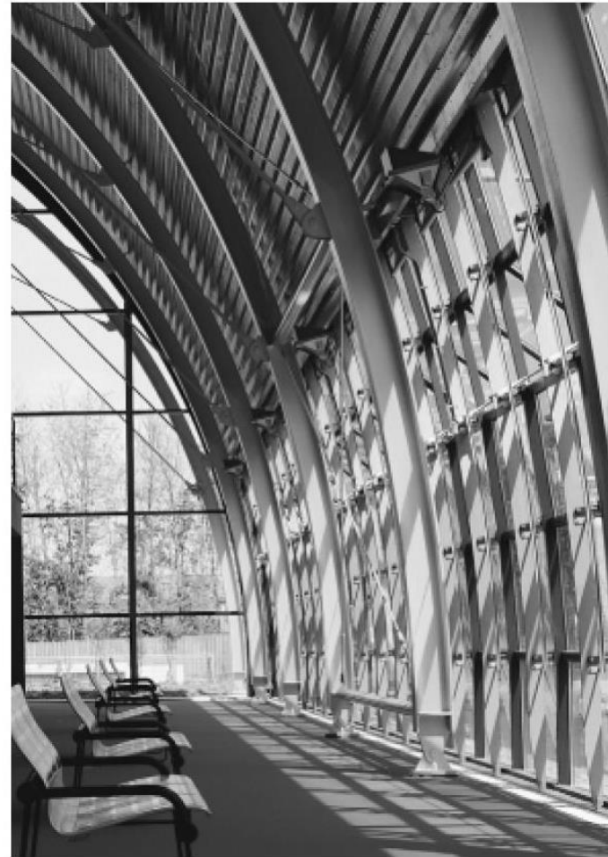
1.4 Thames Valley University, pin-jointed connections supporting curved-arched steel members (architect: Richard Rogers Partnership)
