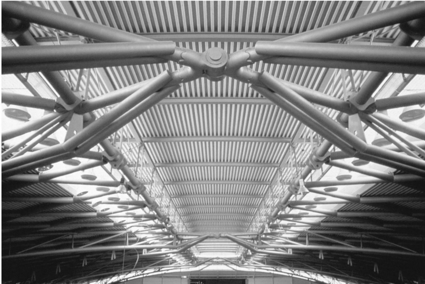
6.14 Pinned connections at Ponds Forge Swimming Pool, Sheffield — see also Colour Plate 20 (architect: FaulknerBrowns)
