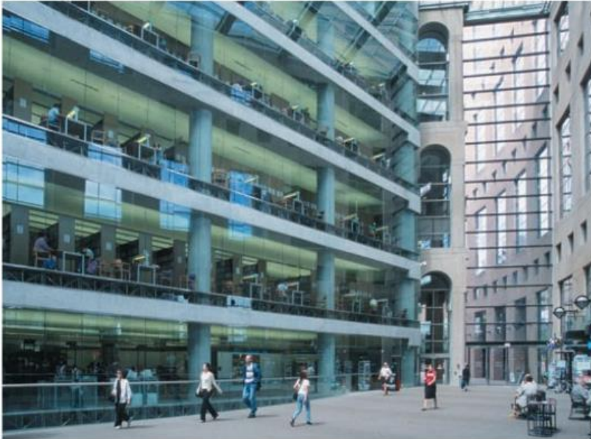
Figure 3.1 Library Square, Vancouver, Canada, Moshe Safdie and Associates Inc., 1995. A typical longitudinal frame and the ends of perimeter transverse
