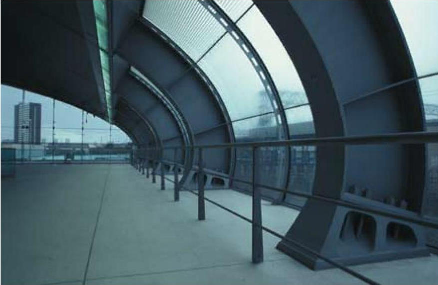
▲ 7.29 Stratford Regional Station, London, England, Wilkinson Eyre, 1999. Curved frames spring from cast-steel bases.
