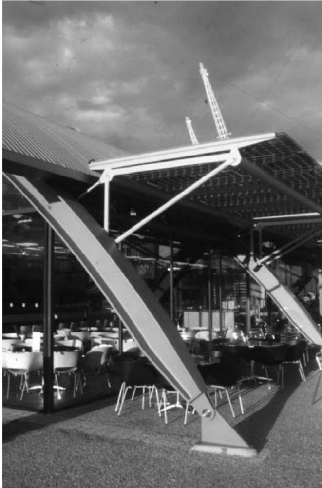
1.3 Pavilion at the Millennium Dome, Greenwich, UK (architect: Richard Rogers Partnership)
