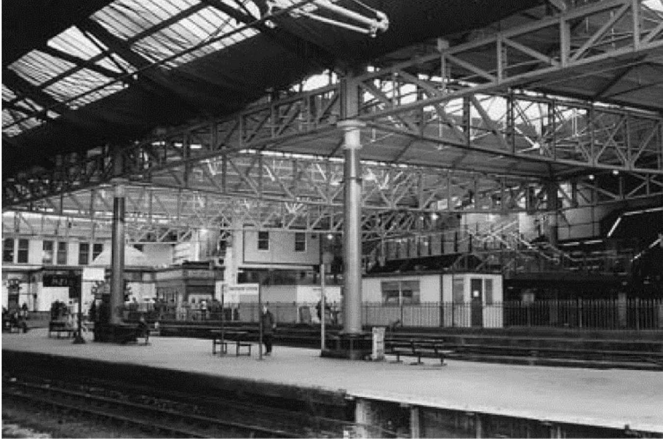
Fig. 12.6 Roof structure, Manchester Victoria station.
