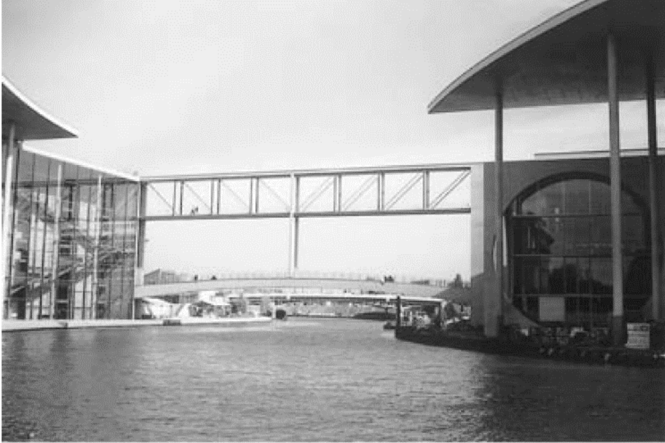
Fig. 12.4 Trussed bridge across River Spree, Berlin.
