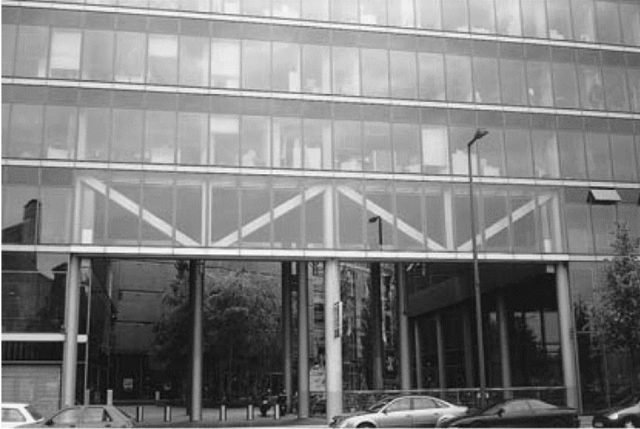
Fig. 12.5 Truss in faade, Sony Centre, Berlin.
