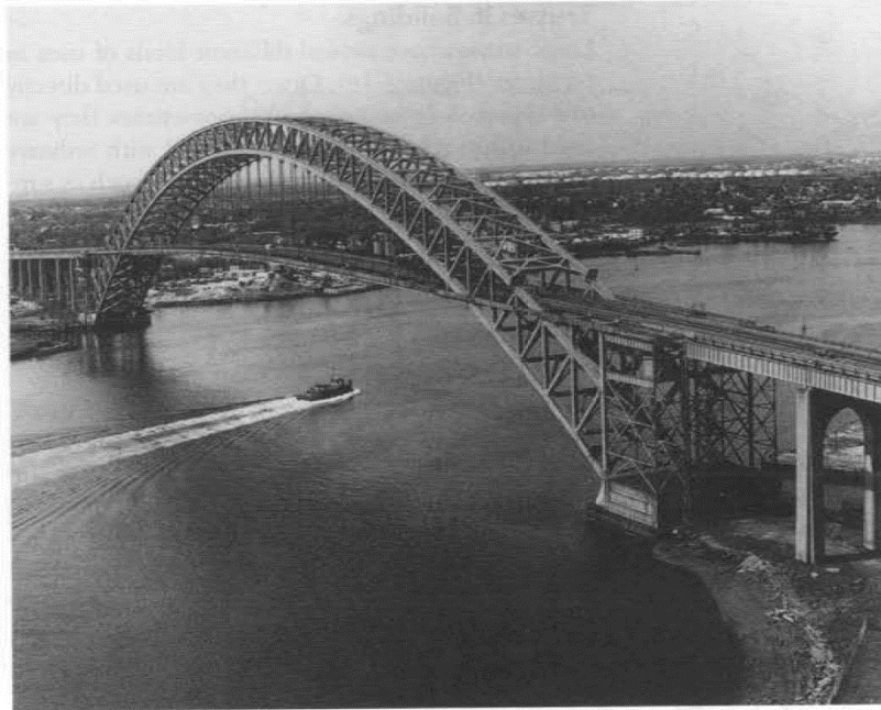
Figure 6.10 The arch of the Bayonne Bridge is restrained from changing shape by its steel trussing, which allows the suspended deck to be very thin. The span is 1,675 ft (520 m). The bridge connects Bayonne, New Jersey, with Staten Island, New York. Engineers: Ammann and Dana.
