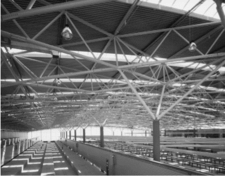
4.40 Stratford Market depot, London (architect: Wilkinson Eyre)
