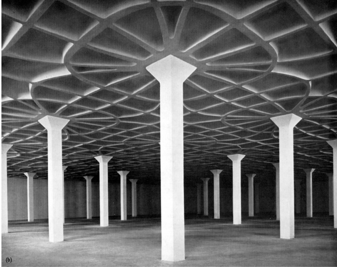
Figure 4.6.7. An experimental concrete floor system designed by Pier Luigi Nervi for the Gatti Wool Factory in Rome (1936). By using custom-shaped pans (of light cement and wire), Nervi was able to re-configure a standard waffle slab so that its ribs followed the lines of static 'flow' from slab to column.
