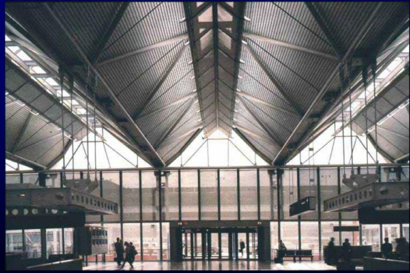
Airport Terminal, Chicago Architect: Helmut Jahn Folded truss
