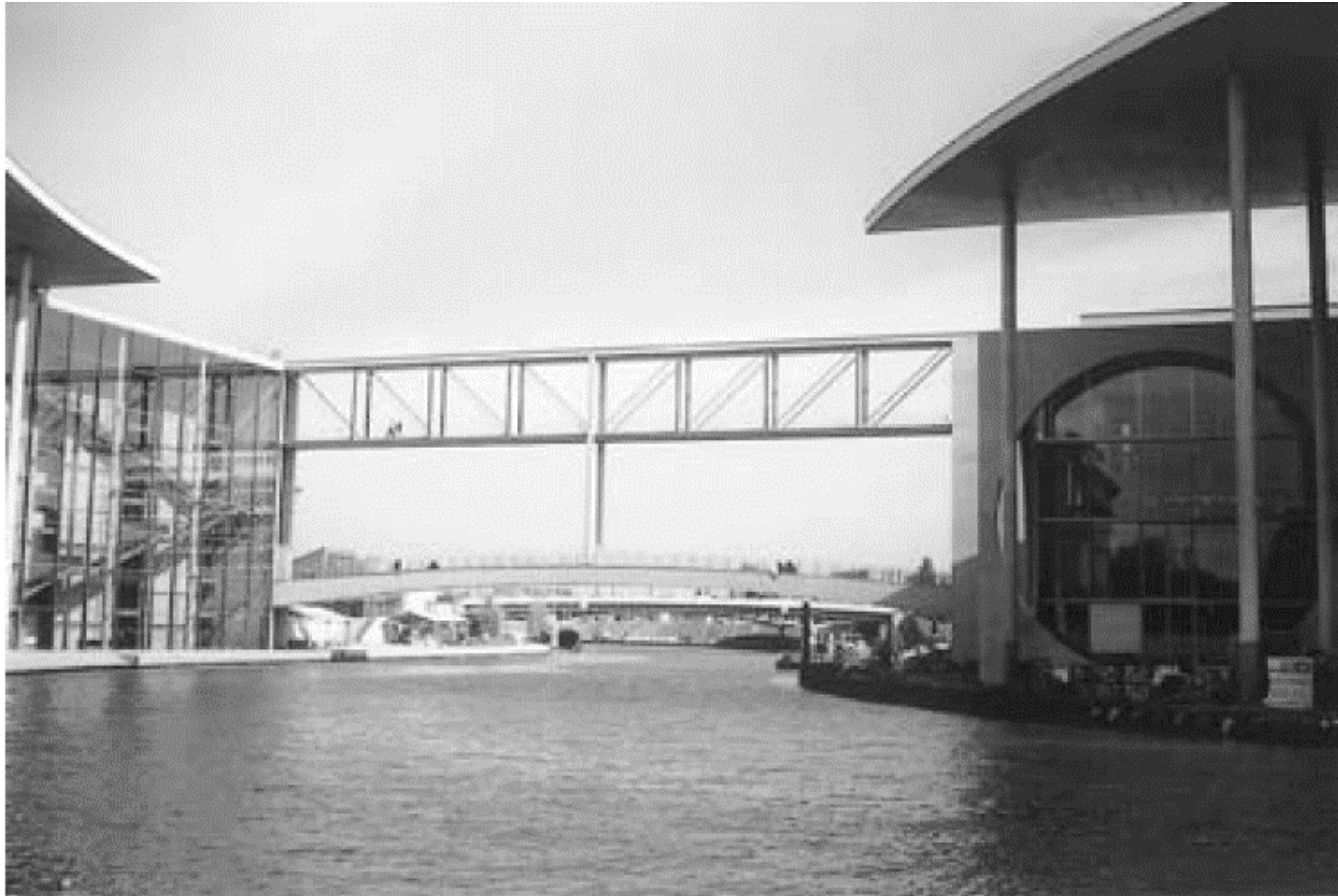
Fig. 12.4 Trussed bridge across River Spree, Berlin.
