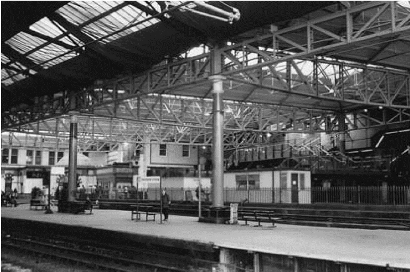
Fig. 12.6 Roof structure, Manchester Victoria station.
