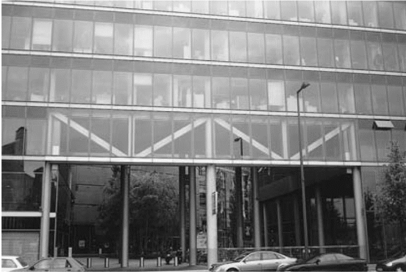
Fig. 12.5 Truss in façade, Sony Centre, Berlin.
