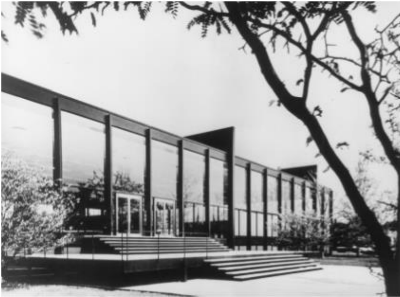
3.4 Crown Hall: external portal frame (architect: Mies van der Rohe)
