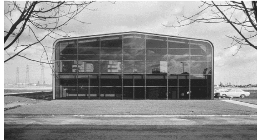
3.7 Portal frame expressed internally behind a glazed-end elevation of a building for Modern Art Glass (architect: Foster and Partners)
