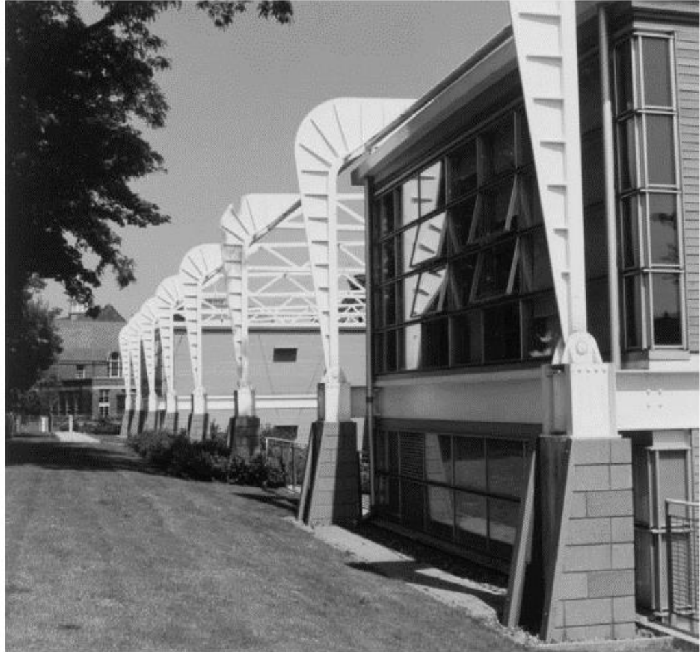
4.33 Lattice girders combine with fabricated steel columns making a hybrid-portal structure at the Brit School, Croydon (architect: Cassidy Taggart)
