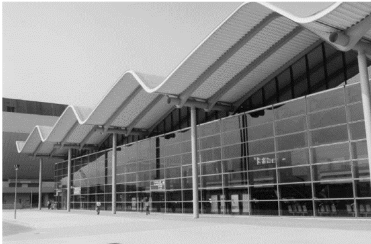
4.23 Tubular columns and spine beams in Hong Kong's Hung Hom Station (architect: Foster and Partners)
