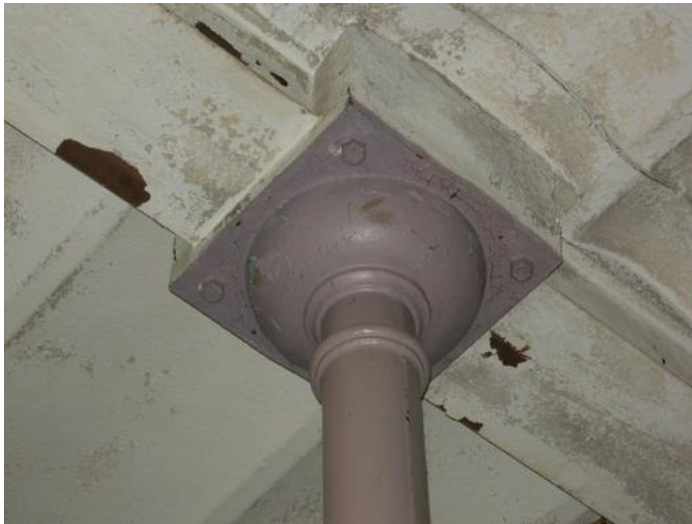
Historical building in İzmir (Masonry walls with interior steel/iron structural system)
