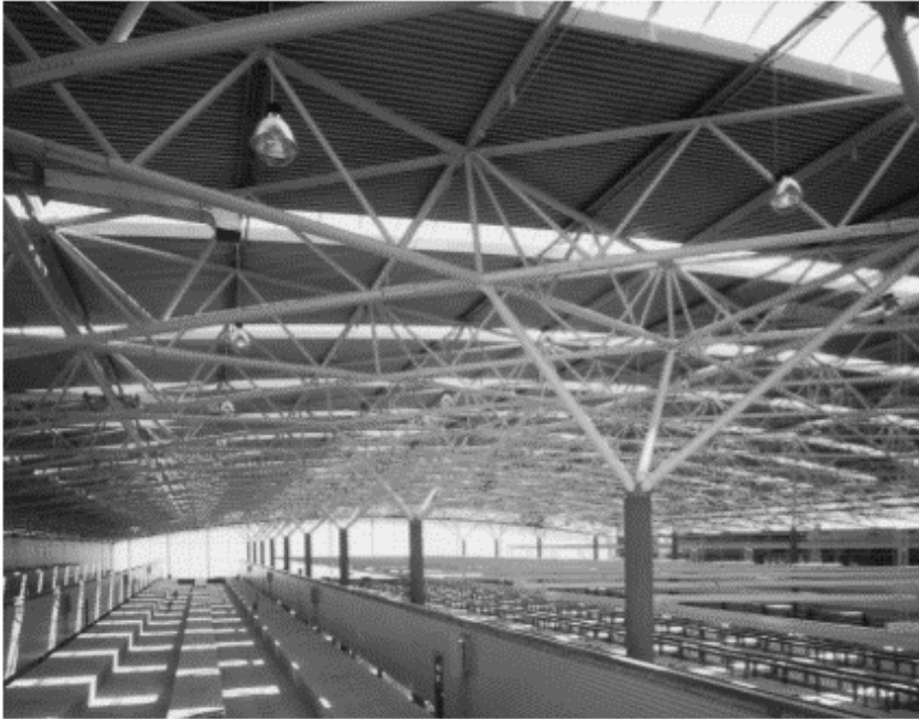
4.40 Stratford Market depot, London (architect: Wilkinson Eyre)
