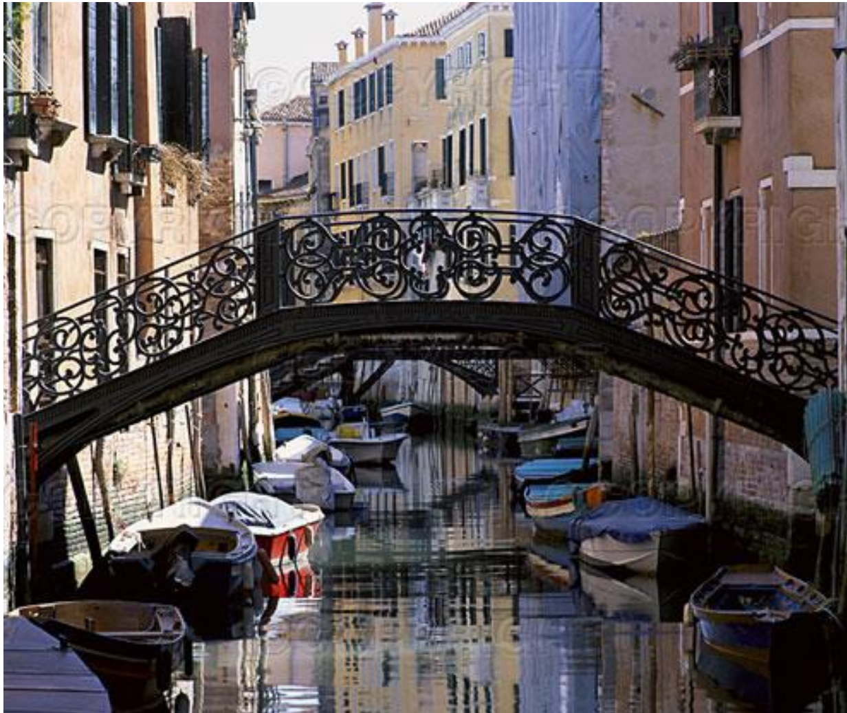
Historical bridges are made of iron/steel in Venice
