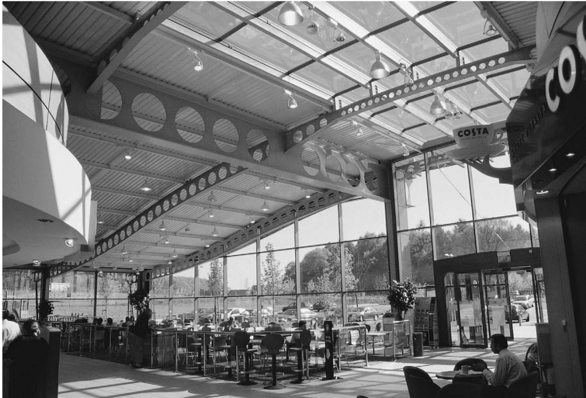
4.2 Curved cellular beam used for architectural effect
