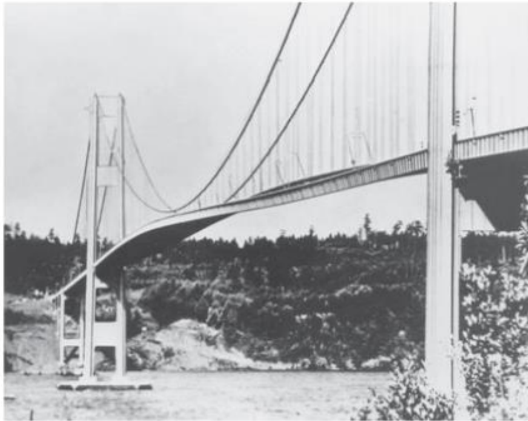
Figure 2.51 An example of nonequilibrium— Tacoma Narrows bridge before collapse.
