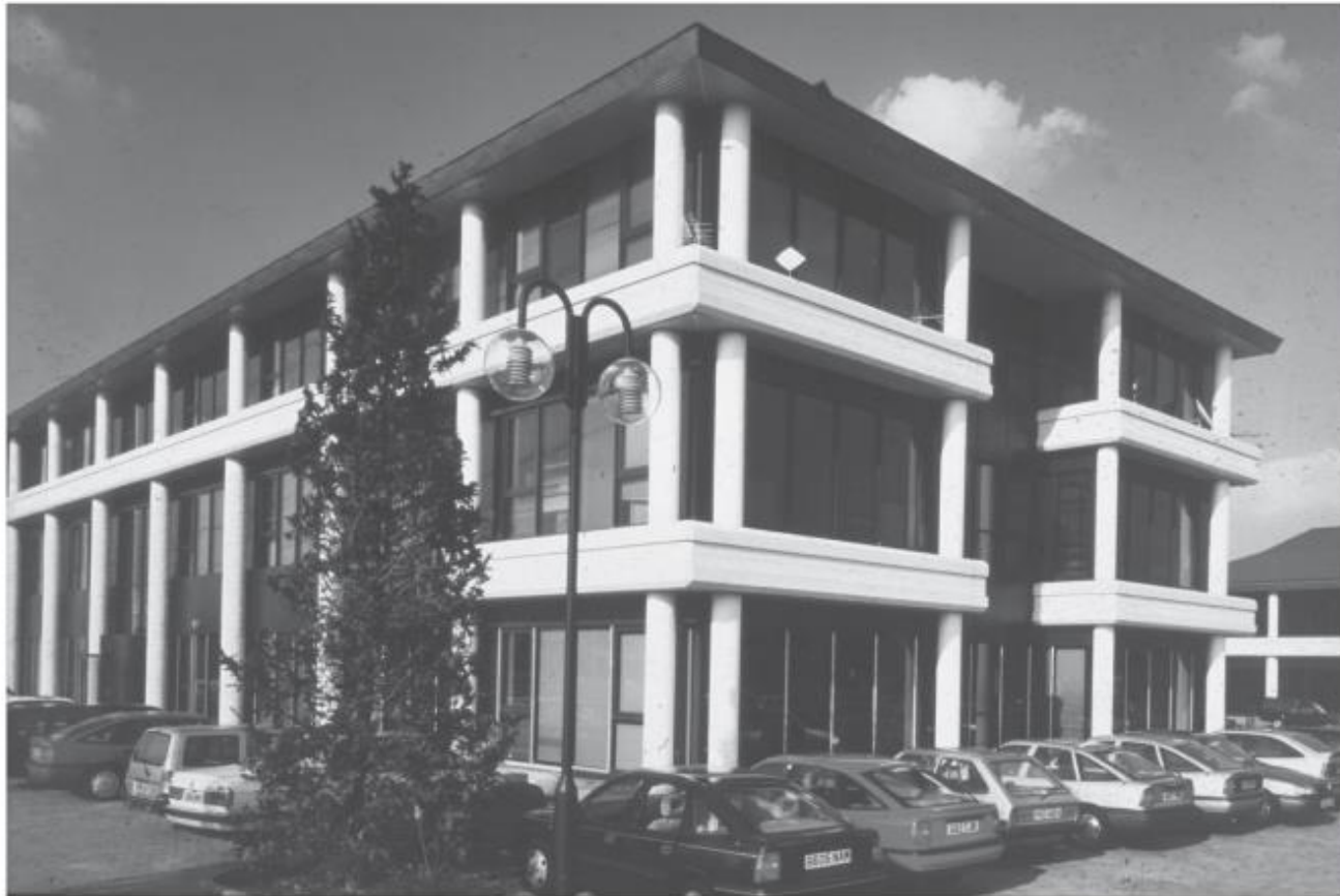
Figure 1.9 Precast 'skeletal' structure with integrated architectural columns and spandrel beams, Reading Business Park. (Courtesy of Trent Concrete Ltd., UK.)
