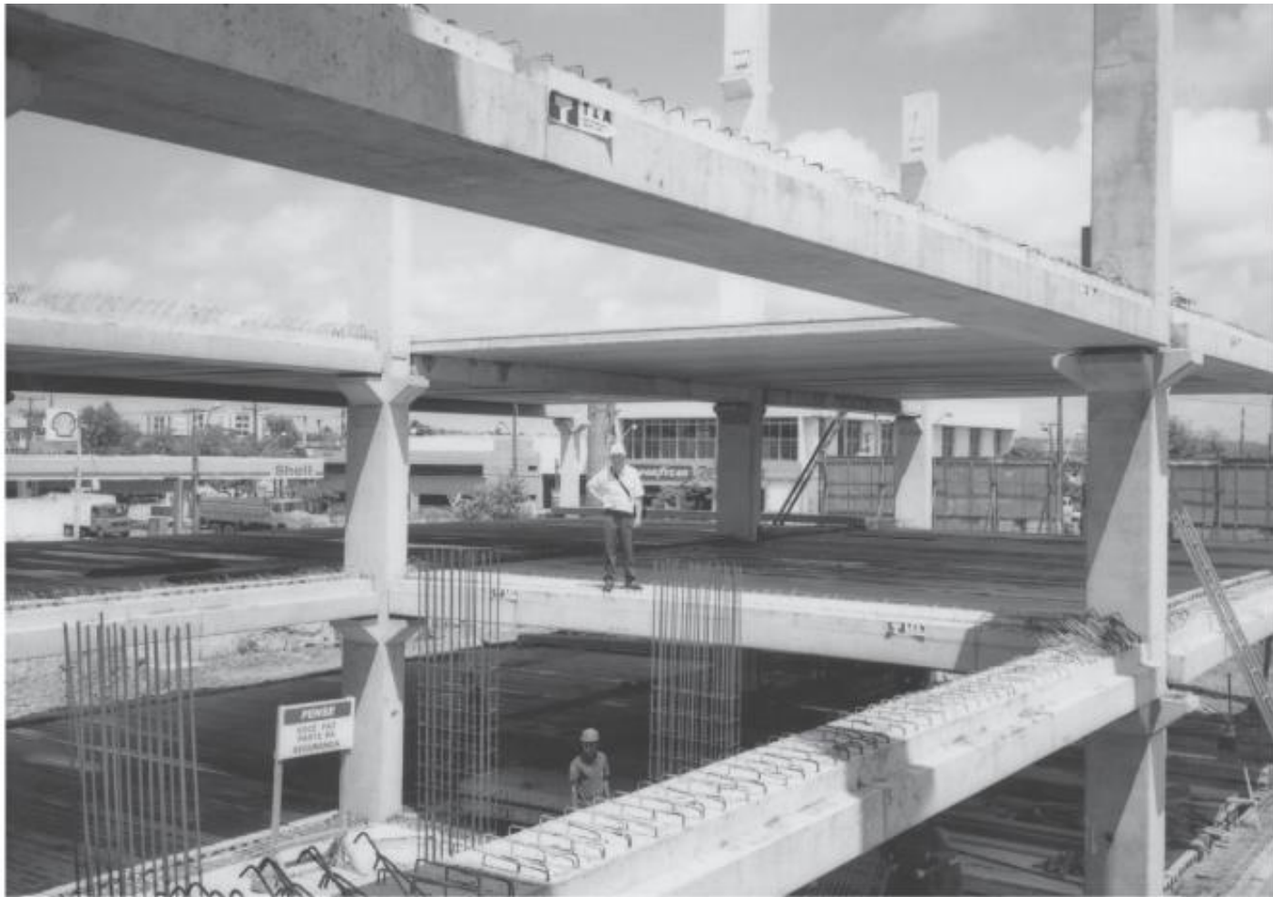
Figure 1.8 Precast concrete 'skeletal' known as 'semi-rigid' frame, Recife University, Brazil.
