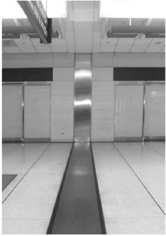
▲ 8.28 A seismic joint between floors, walls and ceilings of two separated structures, San Francisco.
