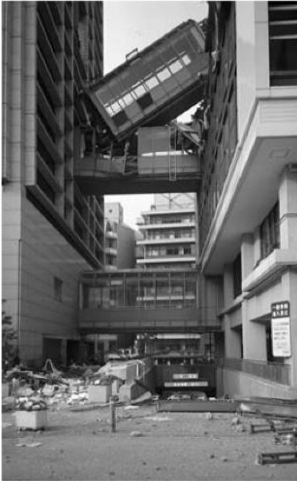
▲ 8.30 Collapsed bridge formerly spanning between two buildings. 1995 Kobe, Japan earthquake.
