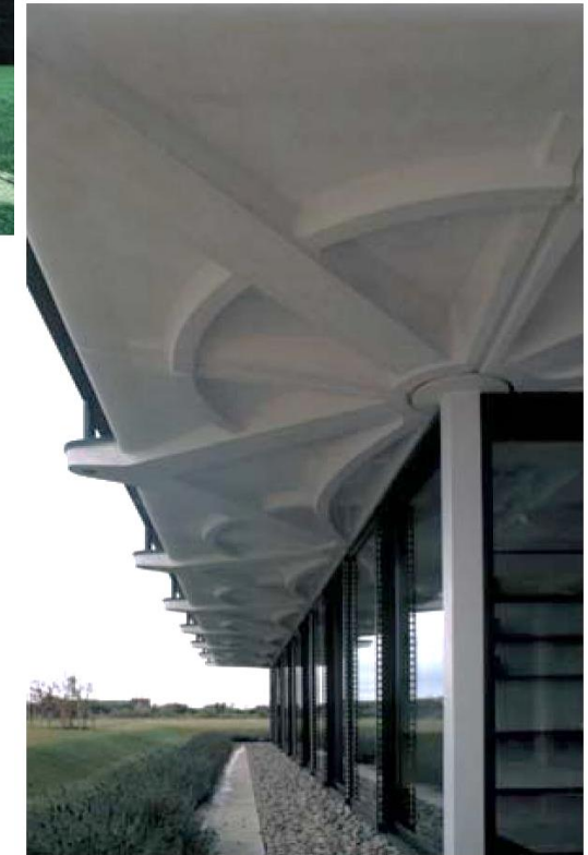
▲ 7.66 Schlumberger Extension building, Cambridge, England, Michael Hopkins and Partners, 1992. Exposed ribbed soffits around the perimeter.
