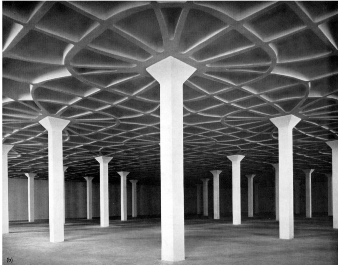
(g) Continuous plate structure with ribs reflecting isostatic lines
