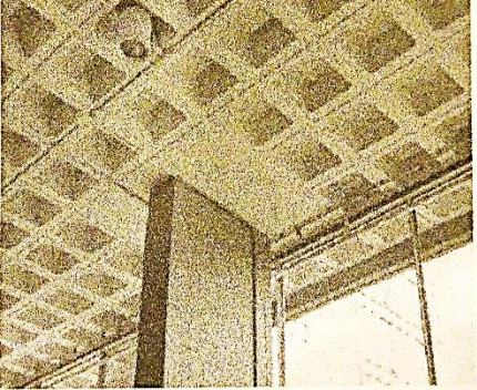
FIGURE 18 A typical waffle slab with infills around columns to increase shear capacity.
