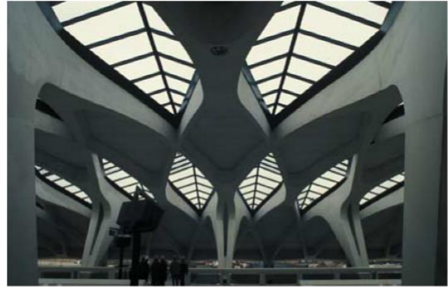
▲ 8.10 A view across the concourse. Glazed areas are integrated with the pattern of ribs.
