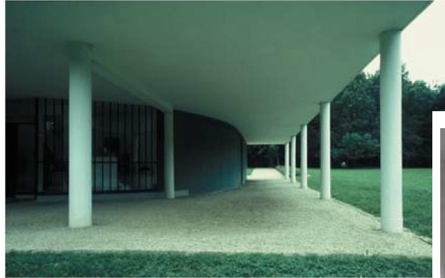
▲ 7.65 Plain exterior column and beam detailing.
