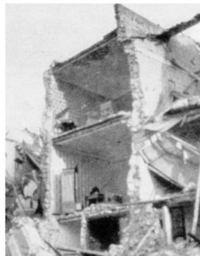
Out-of-plane wall failure
