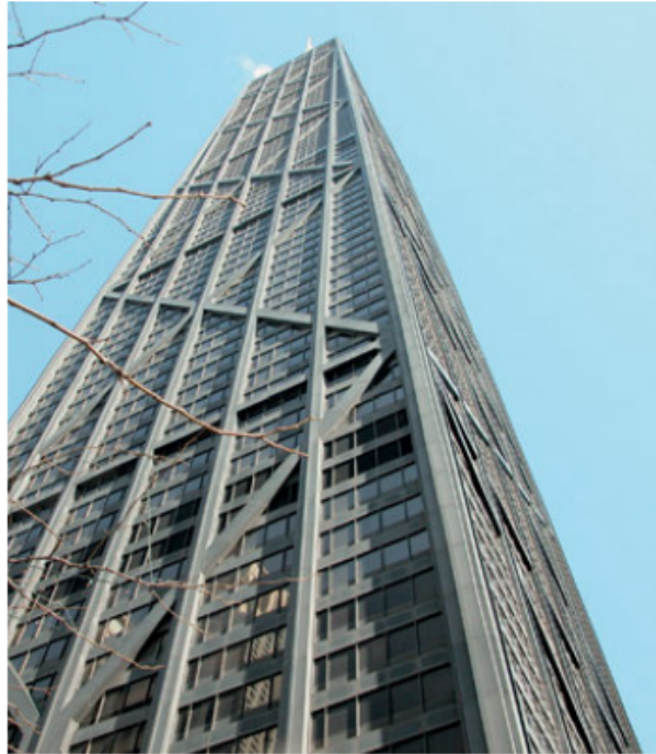
The diagonal braces of the John Hancock Center in Chicago, IL, USA, designed by SOM and completed in 1969, clearly express the lateral bracing system as part of the aesthetic of the façade.
