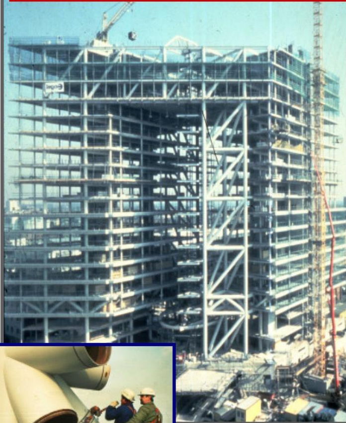
Bracing systems with composite columns
