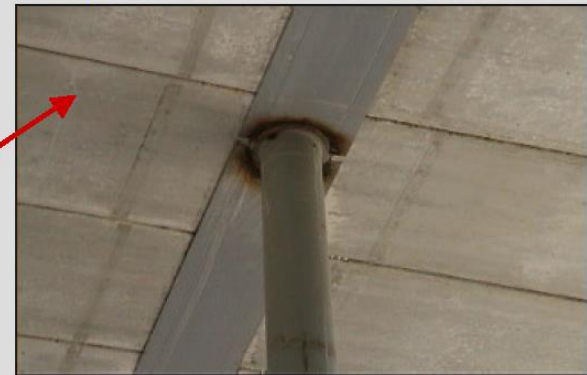
prestressed hollow core slabs
