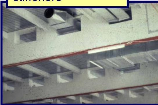
web openings with stiffeners
