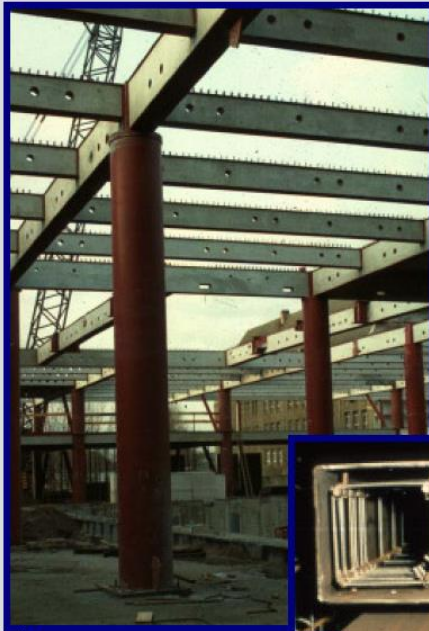
concrete filled hollow sections
