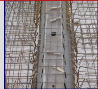
partially prefabricated slabs
