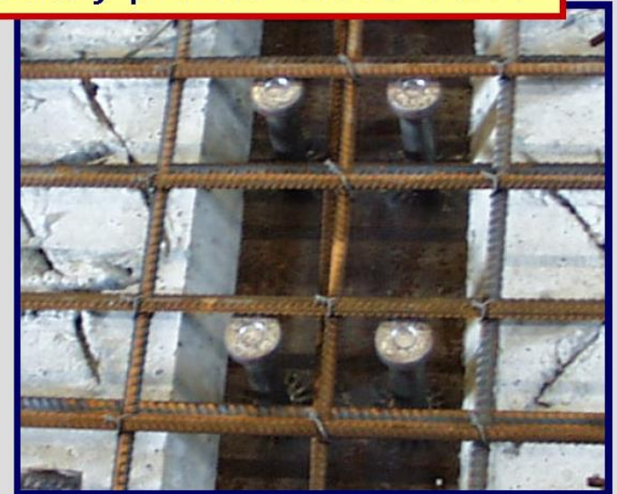
partially prefabricated slabs
