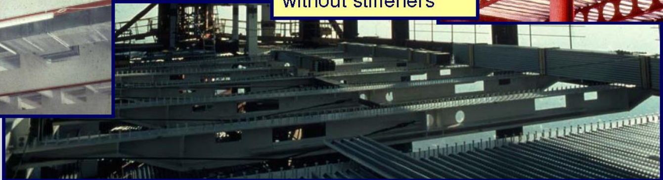
web openings without stiffeners
