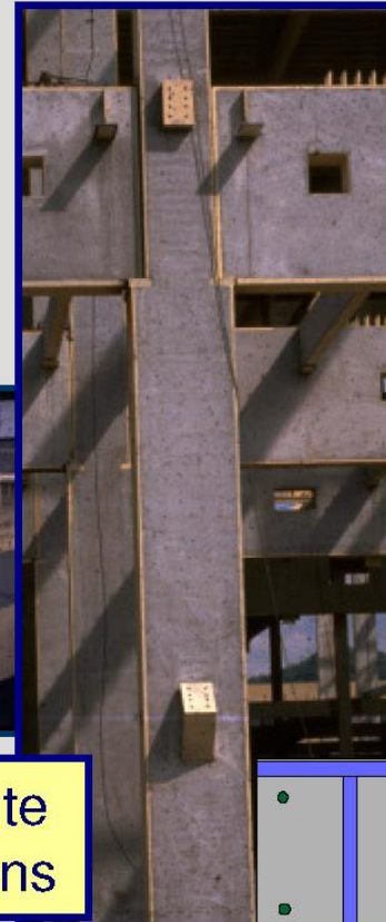
concrete encased sections
