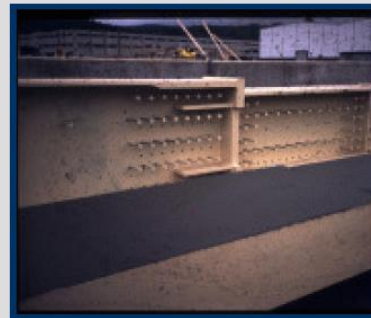
partially concrete encased sections
