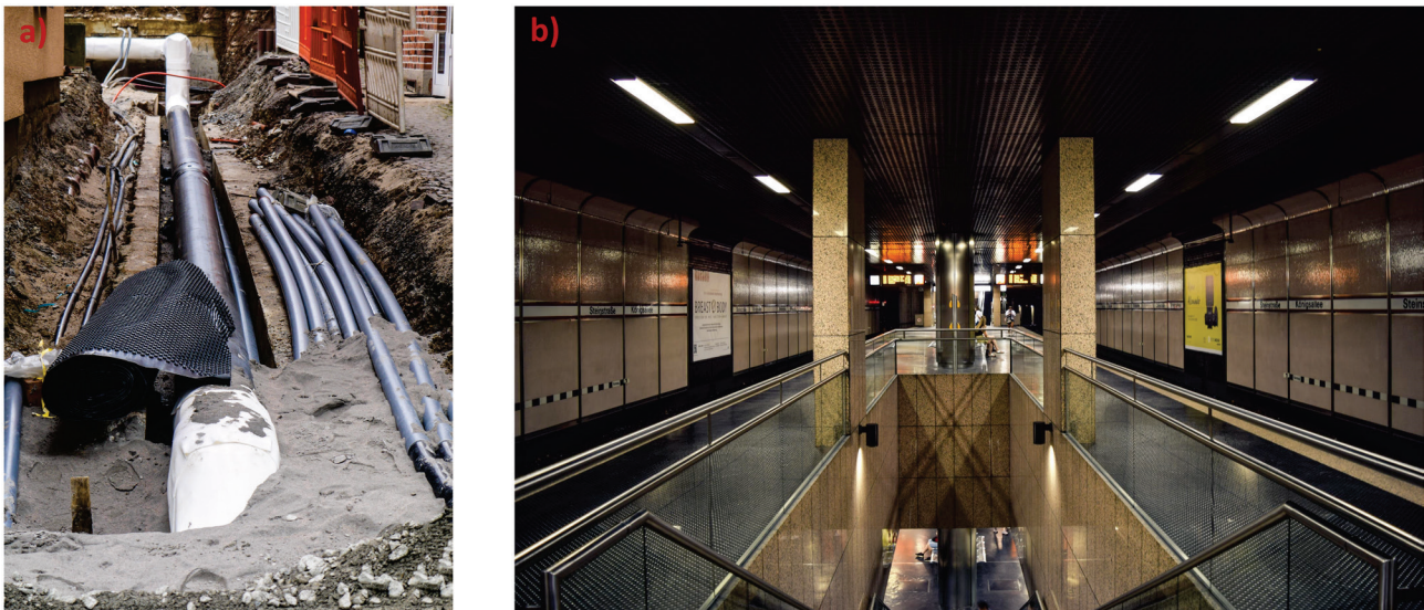
Figure 1. Examples of the underground facilities that legal spaces need to be defined in 3D are (a) underground pipelines, b) storeys of a subway).
