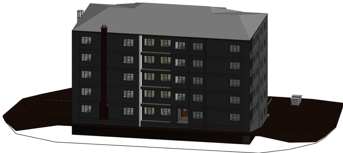
Figure 6. Front view of the building.
