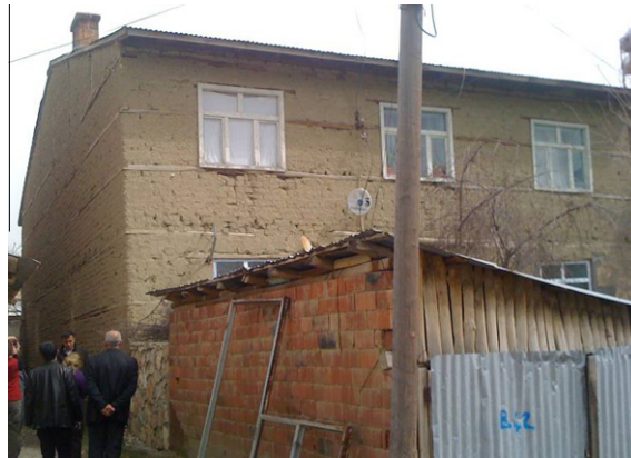
Fig. 30. An example of adobe buildings in Palu.
