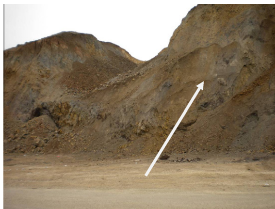
Fig. 12a. Failure surface.
