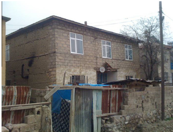
Fig. 17. Typical mixed-type stone-adobe buildings in Palu.
