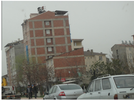
Fig. 16. Typical reinforced concrete frame buildings in Kovancılar.
