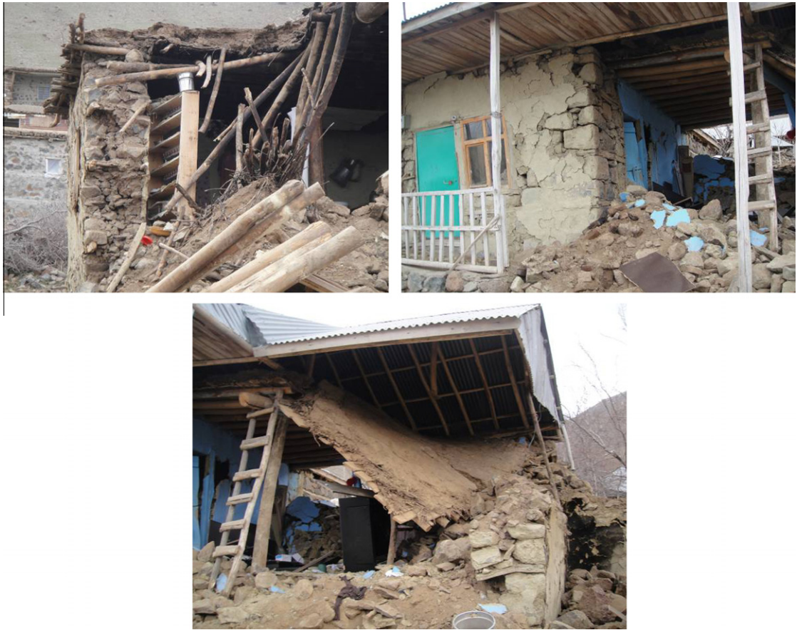
Fig. 20. Typical configurations of stone masonry walls (Göçmezler and Yukarı Demirci villages).
