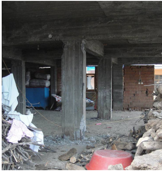
Fig. 31. A reinforced concrete frame building in Yukan Demirci.
