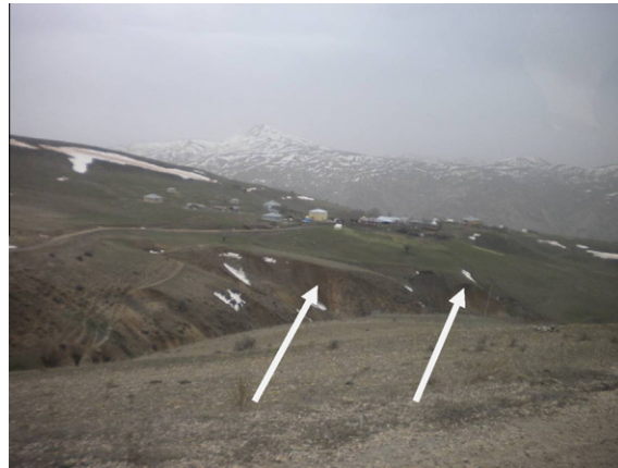
Fig. 12b. Slope failures around the stream in the region.
