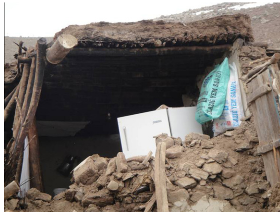
Fig. 21. Heavy compacted clay roofs (Göçmezler village).
