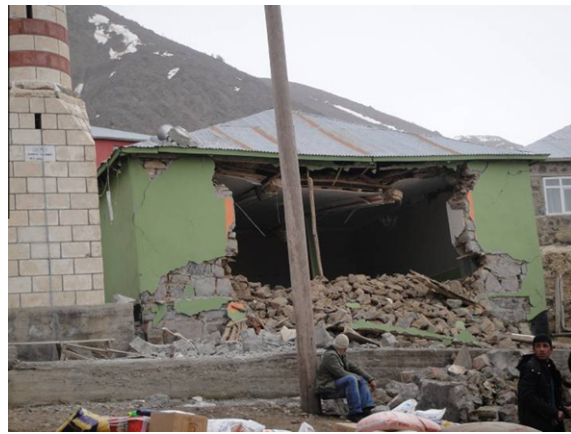
Fig. 23. Excessive wall lengths without any lateral support or restraints and large openings (Yukarı Demirci village).
