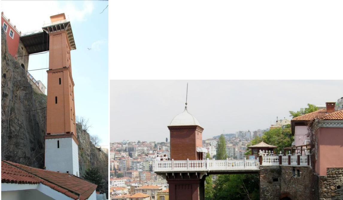
Figure 3. Asansor Tower and terrace view
