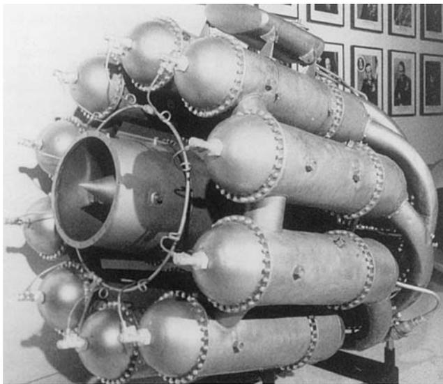
Figure 48. Combustor and Jet Pipe of Whittle W.IX Engine.
