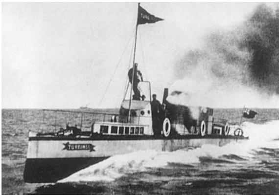
Figure 21. The 34 Knot "Turbinia" at Spithead Naval Review in 1897—First Demonstration of Steam Turbine Propulsion. (Parsons, 1926)
