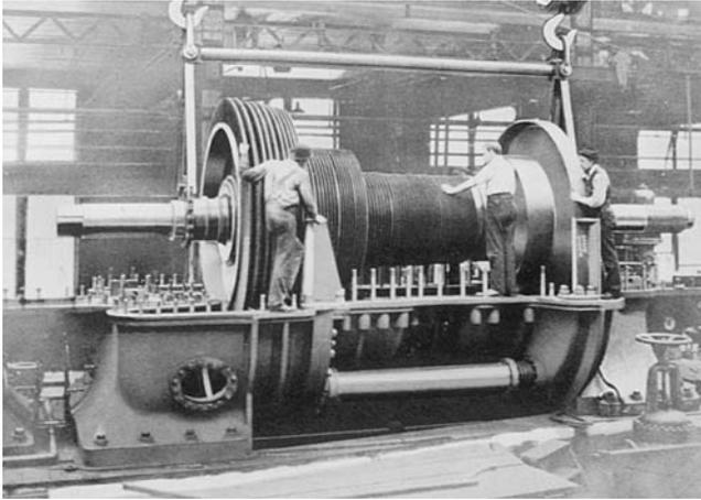
Figure 19. Parsons Axial Flow Steam Turbine Opened for Inspection. (Parsons, 1926)
