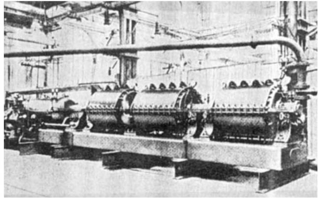
Figure 29. Gas Turbine Developed by Lemale and Armengaud, Circa 1905, Three Centrifugal Compressor Cases (25 Impellers) Designed by Rateau. (The turbine wheel diameter was 37 inches.) (Stodola, 1927)
