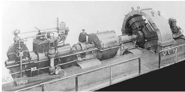
Figure 20. Photo of Parsons Turboalternator. (French, 1908)
