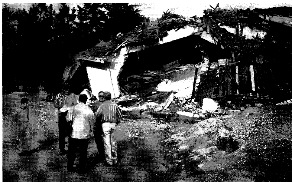
Figure 2.26. Fault rupture extended beneath the music building of a primary school in Kullar, about 4 km east of Izmit Bay. About 2 meters of lateral offset and 0.5 meter of vertical offset caused partial collapse of the school.
