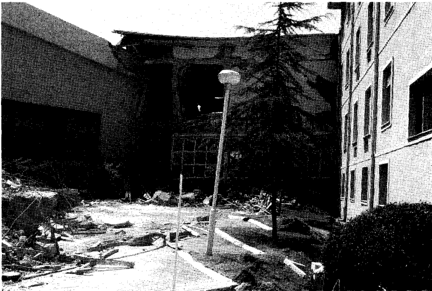
Figure 2.17. Fault rupture between and through a complex of three-story buildings, west part of Gölçük Naval Base.
