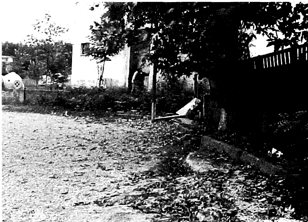
Figure 2.27. Fault rupture extended toward and went around a two-story concrete frame building near the damaged school in Kullar shown in figure 2.26. Approximately 1 meter of lateral offset extended to, but was arrested at, the building. Slip on the fault strand was transferred to an adjoining parallel fault strand.
