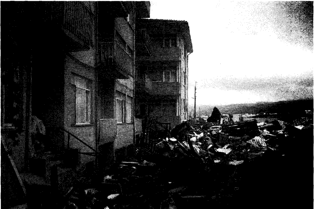
Figure 2.14. Four-story apartment house that collapsed from surface rupture on right side of photo, west of Gölcük Naval Base. Fault rupture passes left to right across the middle of the photo between two standing apartment buildings. These apartment buildings were originally aligned and are now offset about 4 meters relative to one another across the fault.
