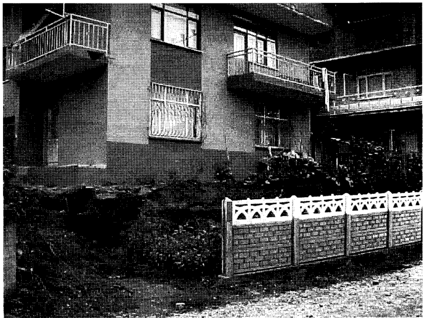
Figure 2.36. Two-story house in the city of Gölcük with 1.5-meter fault scarp. The house was not damaged.
