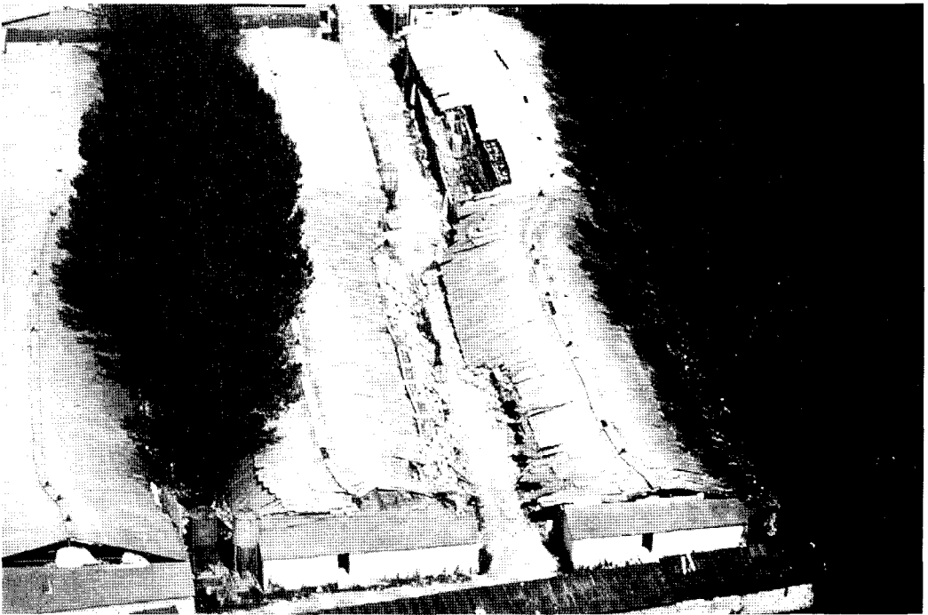
Figure 2.33. Directly east of Arifiye, surface rupture of about 5 meters on the Sakarya fault segment caused partial collapse of three agriculture warehouses.
