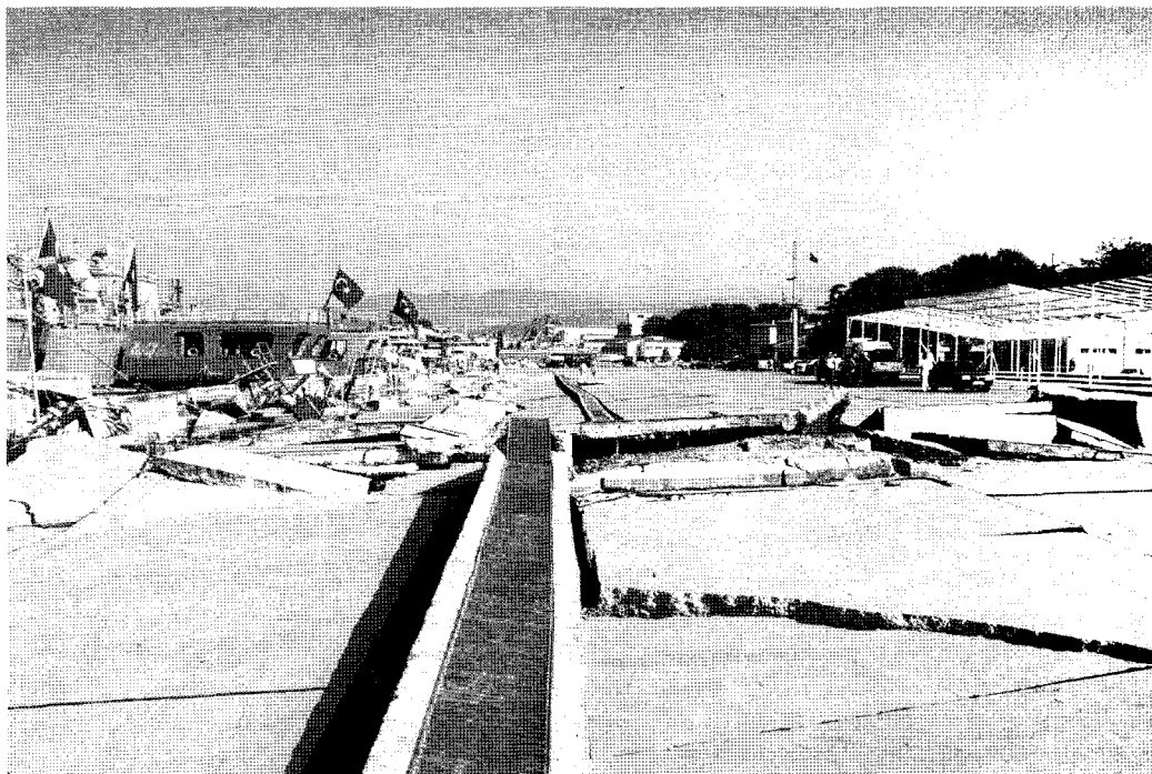
Figure 2.21. Fault offset of about 2 meters of a dock at the Gölcük Naval Base.
