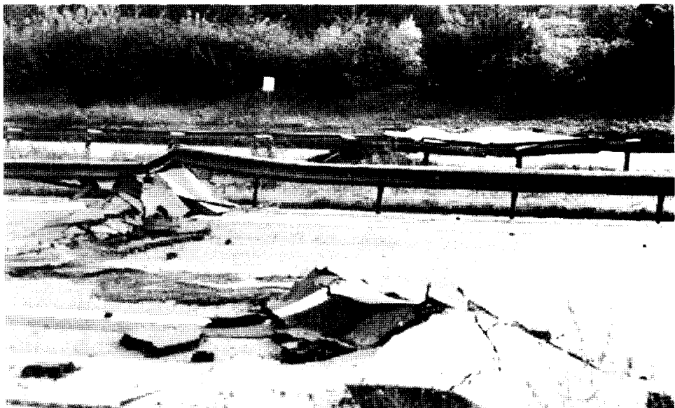
Figure 2.38. Fault offset of about 3 meters along the Sakarya fault segment near the town of Arifiye damaged roadways and the Trans-European Motorway.
