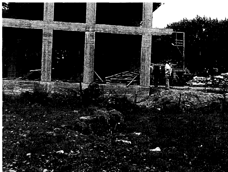
Figure 2.28. Four-story concrete frame building under construction in eastern Kullar City. Fault rupture extended beneath the building, but the building foundation decoupled from soil, and the structure was not damaged.
