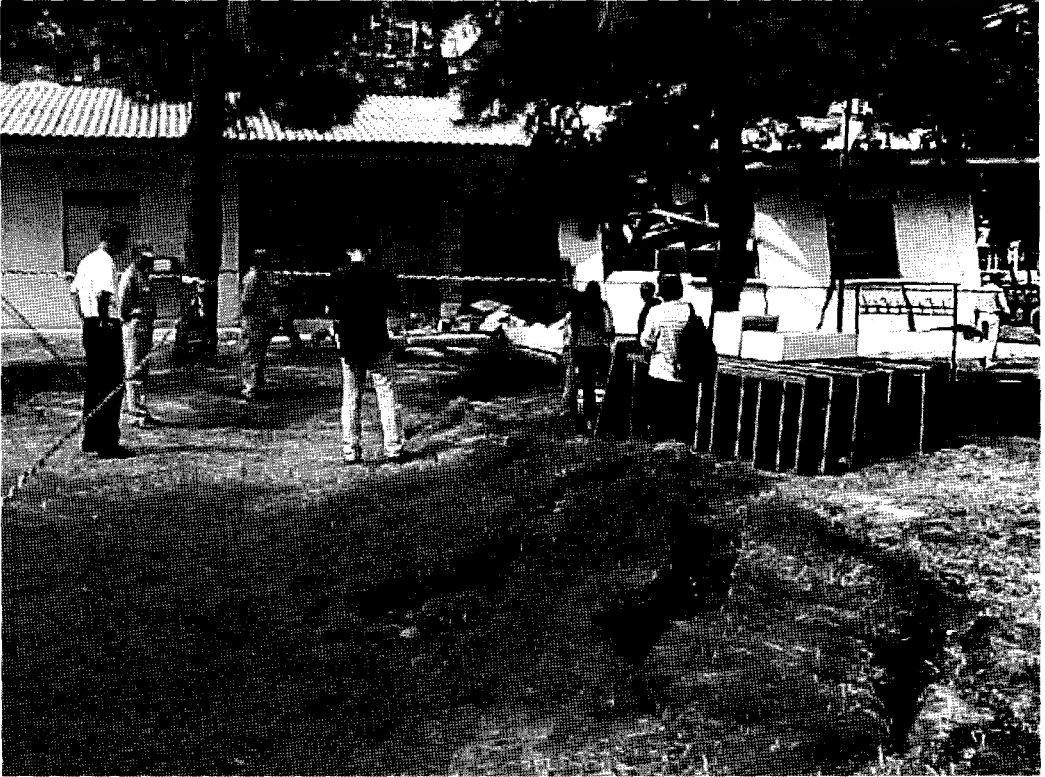
Figure 2.16. Fault rupture through single-story building, west part of Gölçük Naval Base.
