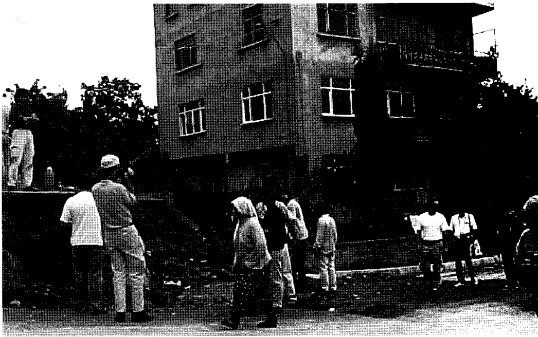
Figure 2.35. Normal fault displacement of 2.4 meters passed within 1 meter of a four-story concrete frame apartment building. The building is undamaged.
