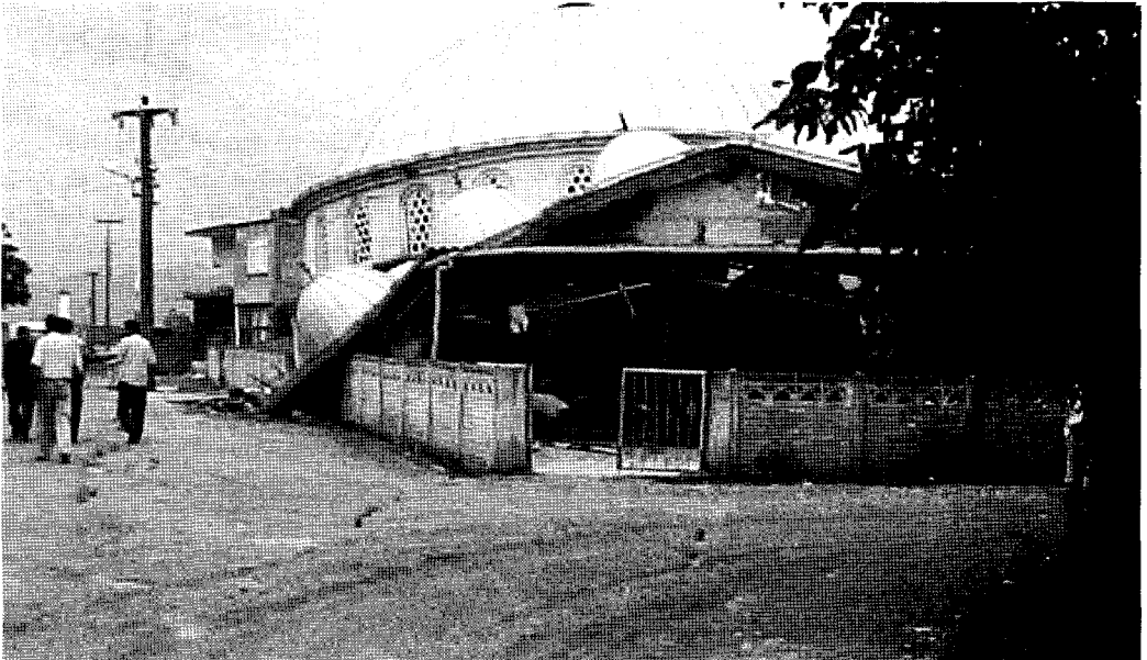
Figure 2.24. Vertical surface displacement of about 1 meter extended beneath and caused collapse of a mosque in a residential area directly east of the city of Gölcük.
