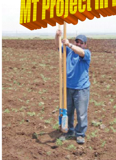
Volkan Tuncer digging a vertical coil hole
