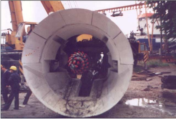
Fig. 2. General view of the roadheader used in the Hereke Tunnel.
