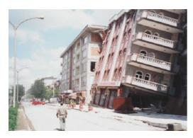
Liquefaction induced bearing capacity failure of a building after Adapazari EQ, 1999
