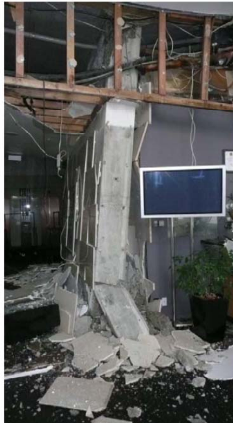
FAILURE OF SHEAR WALLS
