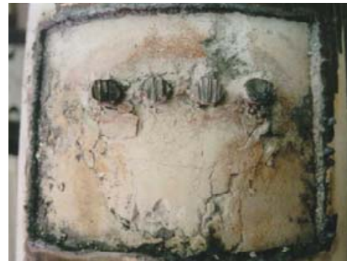
CONCRETE ANCHORAGE FAILURE
