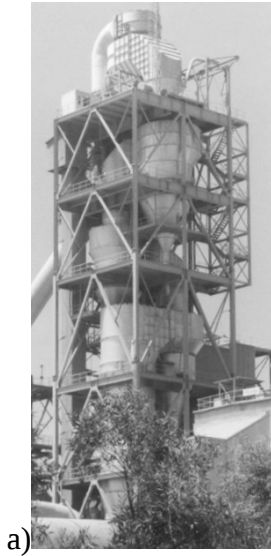
Fig.1 The pre-heater tower and a typical vibration spectrum in rms on the top platform. (North-South, Capacity 130 tons/hour)
