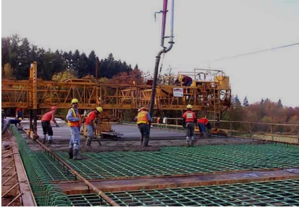
Bridge deck constructed with epoxy-coated reinforcing bars
